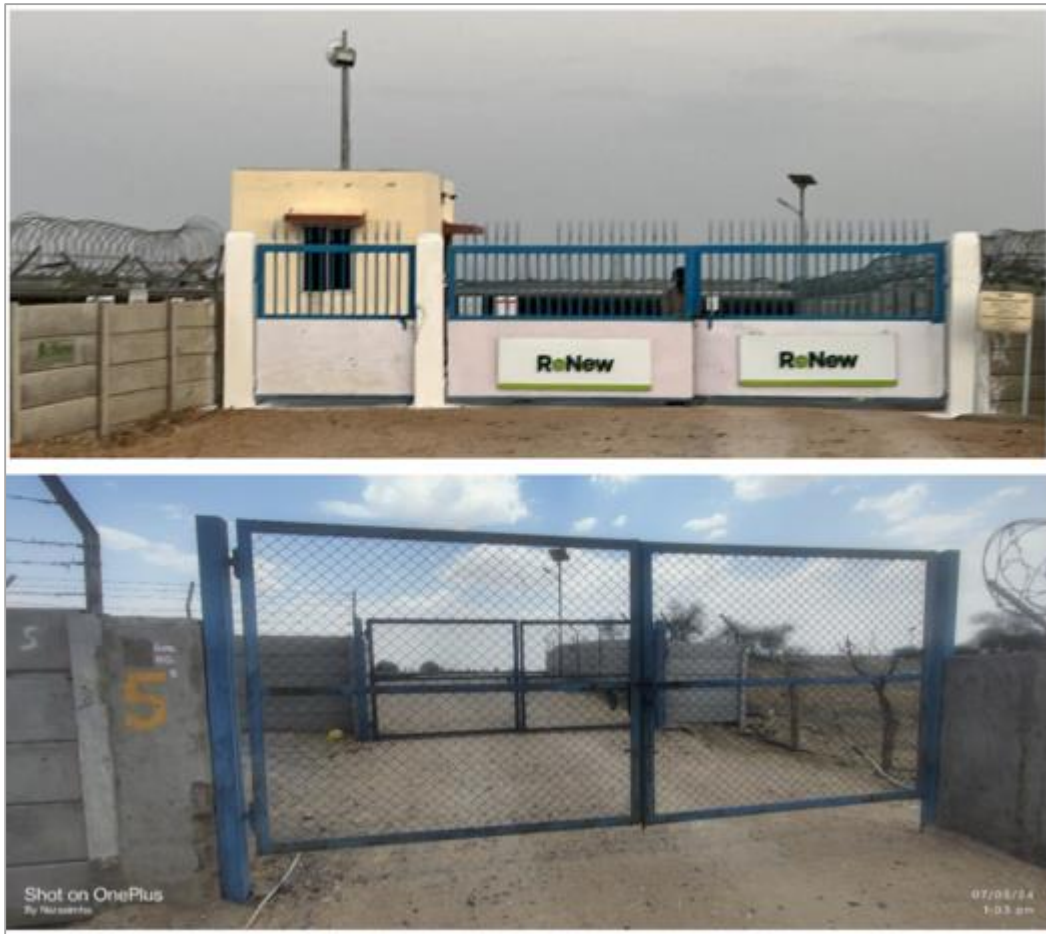
Figure 0-2: Entrance to the project Site
